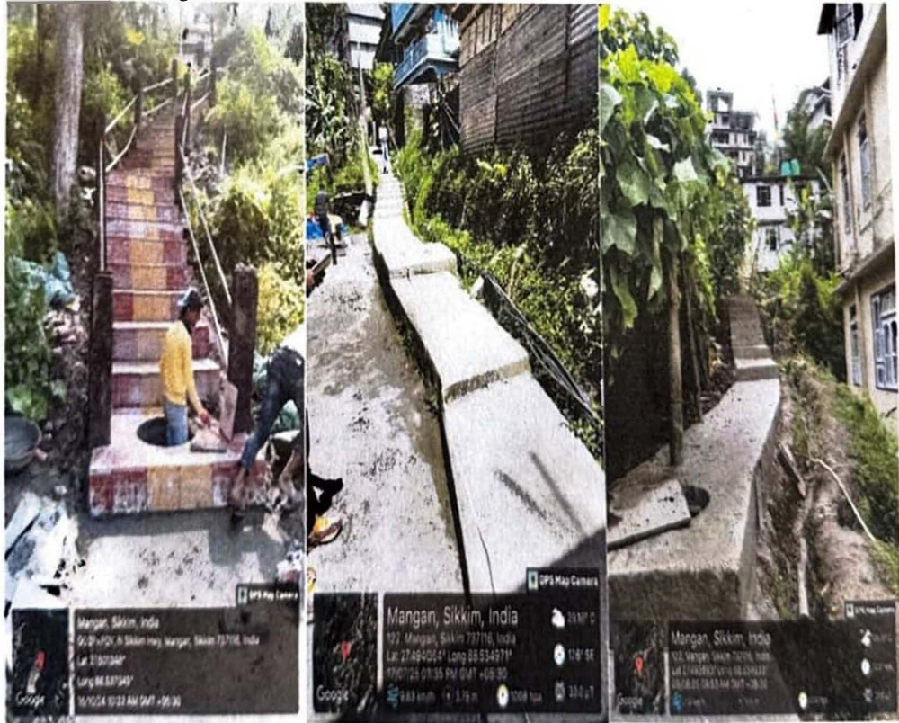
Restoration of Footpath post laying of sewer lines along DC Quarter footpath, Pentok footpath and Upper Singhik footpath in Mangan
