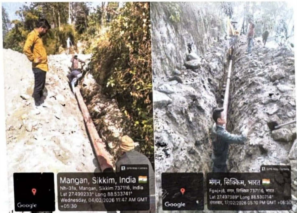
Laying of DI pipes along BAC Sankalang bypass road and PMGSY road in Mangan
