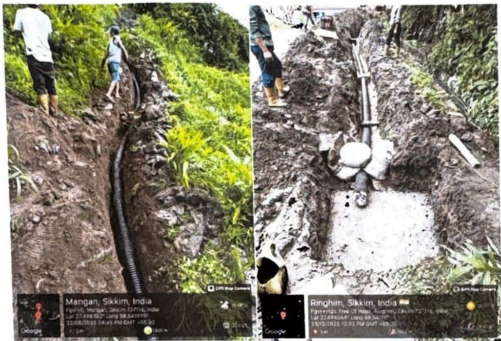
Laying of DWC pipes above Power colony area and Ringhim in Mangan
