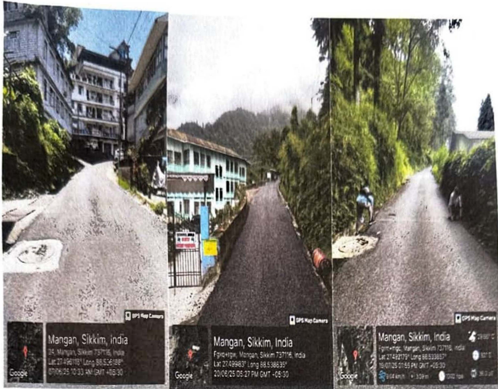
Restoration of road post laying of sewer lines along DAC road, Zilla Bhawan road, Pentok and Mangan school road in Mangan
