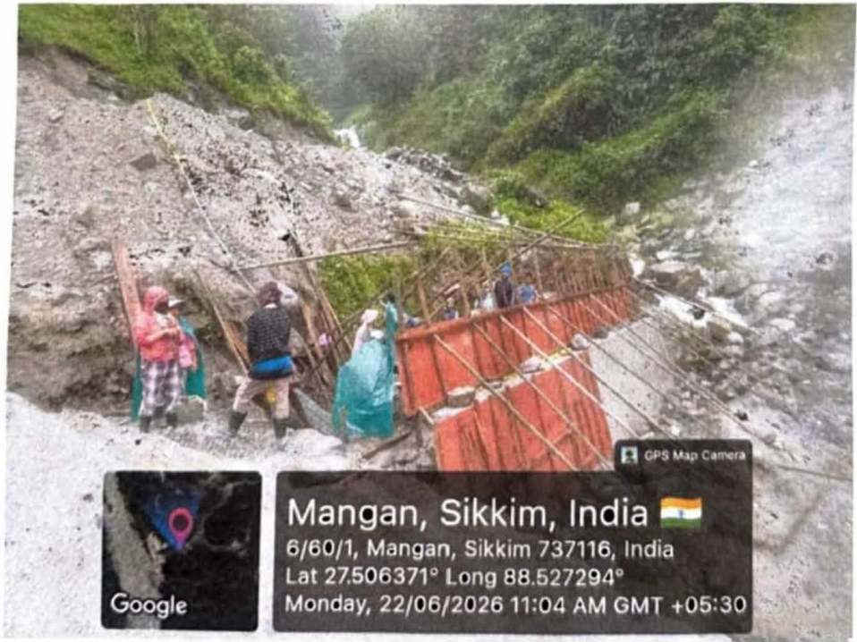
STP site levelling work for Mangan Sewerage System
